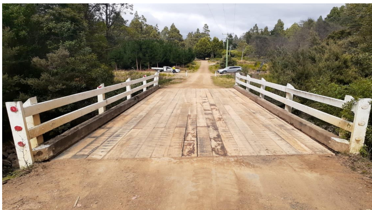
Barretts Road Bridge (Humboldt River) after re-decking
