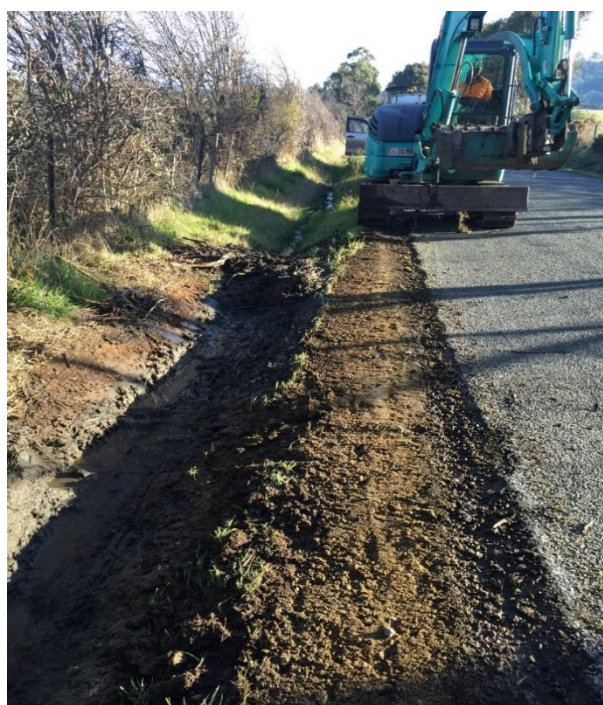
Clearing table drain on Glenfern Road
