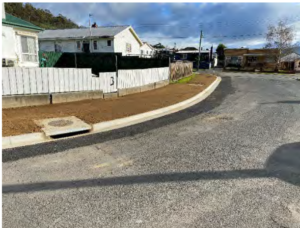
Figure 9 - New Kerb and Gutter, Stormwater Pipe and Sub-soil drainage in Andrew Street, New Norfolk
