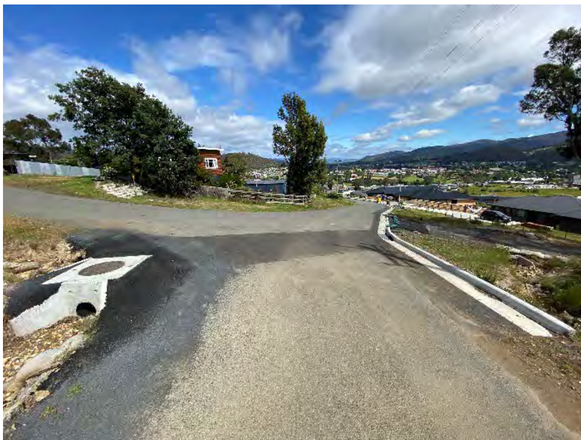
Figure 10 - New Kerb and Gutter and Stormwater at Poulter's Road, New Norfolk
