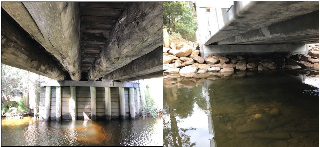
Figure 1 Junee Road bridge timber beams replaced with concrete beams
