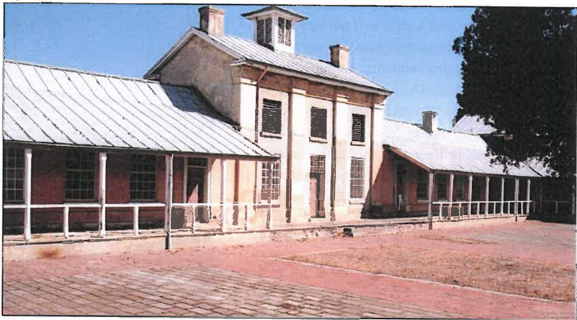
The Barracks; part of the historic Willow Court precinct. Work is currently underway to restore this historic site.
