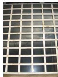
Windows, 'C' Ward
